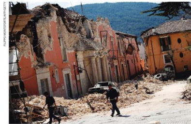
More than 300 people perished in the earthquake that struck the medieval centre of L'Aquila.
